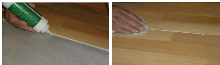
Beauflor Seam Bond application and clean up with a damp cloth
