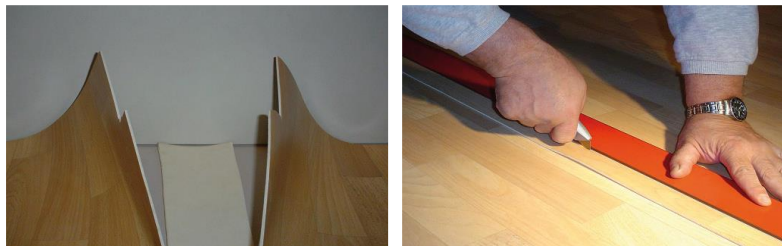
Scrap piece placed under the seam - double cut with a straight edge
